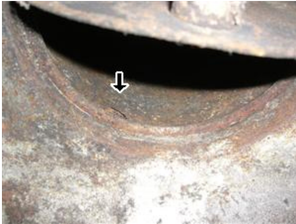
4.1 Picture 1 Hole in flue
