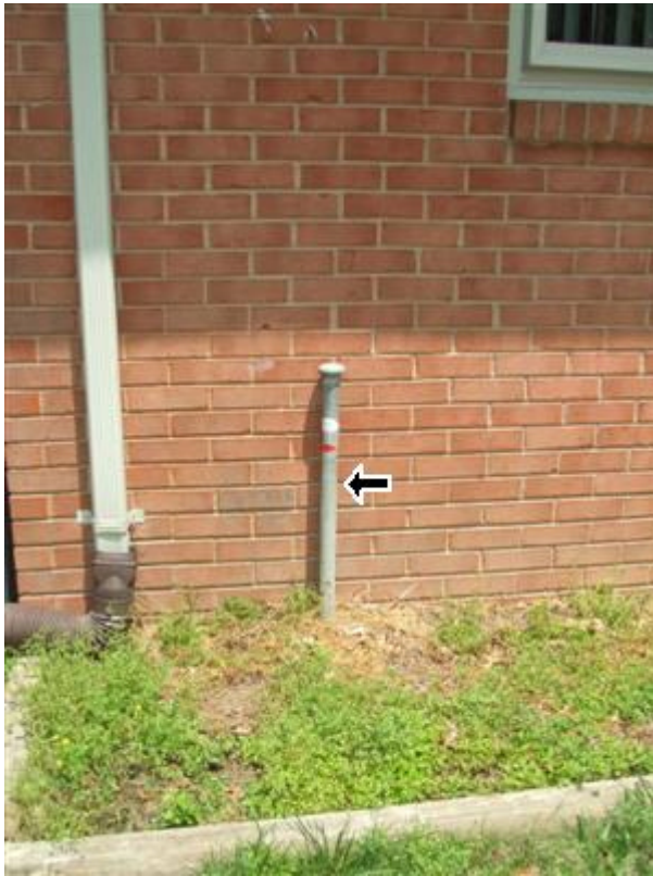
2.4 Picture 1 Oil tank vent
