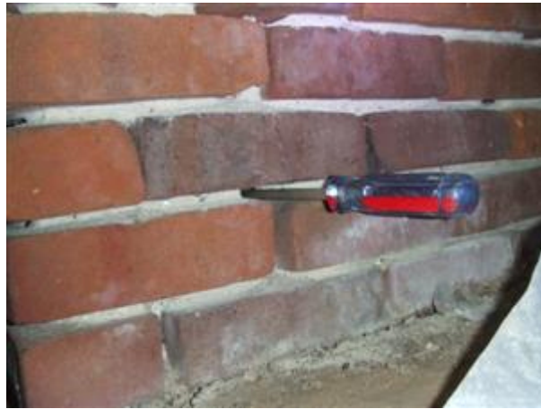
11.0 Picture 2 Screw driver 6" into soft mortar
