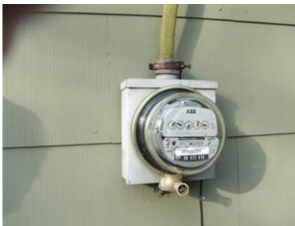
8.0 Picture 4 Meterbase rated for 100 Amps
