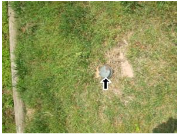
2.4 Picture 2 Oil tank fill cap
