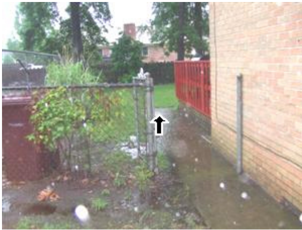
5.5 Picture 2 Standing water 2" deep on walkway
