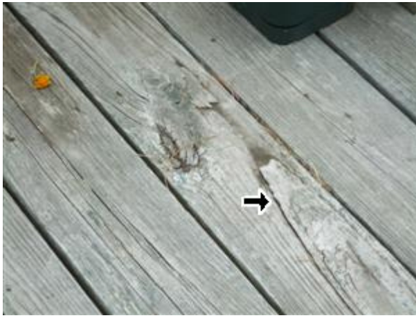
5.4 Picture 2 Splintered board
