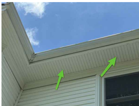
Soffit ventilation
