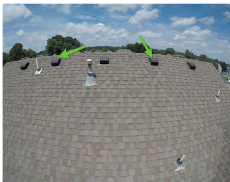
Static outlet vents
