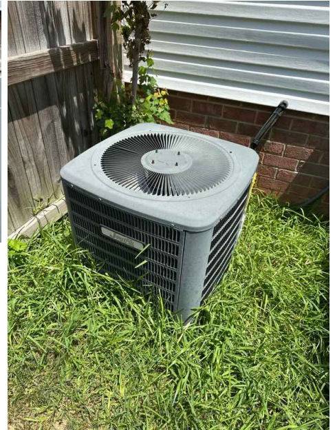
Upstairs AC condenser, 2 ton, r410a , MFG. 2010
