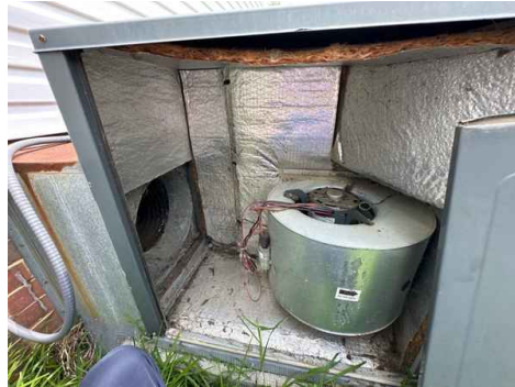
Downstairs package unit blower compartment
