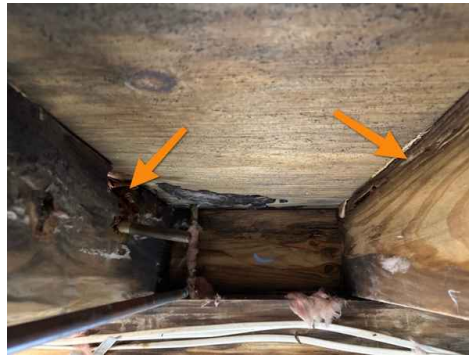
2 joists damaged under kitchen sink
