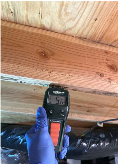
5% moisture very dry well below average, satisfactory
