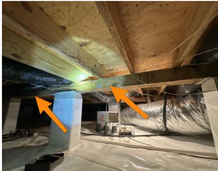
Under front entryway, gutter beams marked with X for repair, no damages
